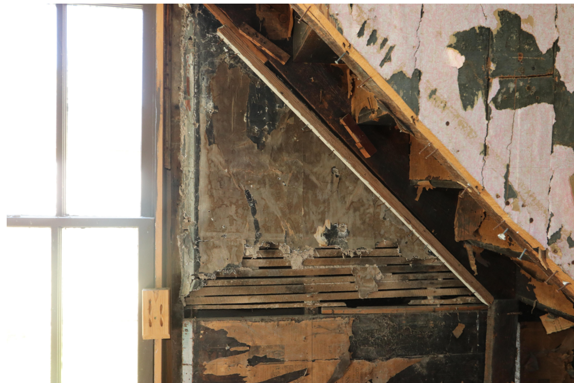
DETAIL OF HISTORIC PLASTER AREA UNDER STAIR TO BE PROTECTED NOT TO SCALE
